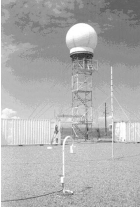
Figure 1 The MIT 5-cm (C-band) research radar deployed in Albuquerque, New Mexico. The nearly spherical radome protects the radar antenna and sits on top of a tower that places the antenna above blocking objects. The transmitter, receiver, and operating consoles are located in the buildings below the tower. (Photo courtesy of MIT Weather Radar Lab, D. Boccippio.) See ftp site for color image.
