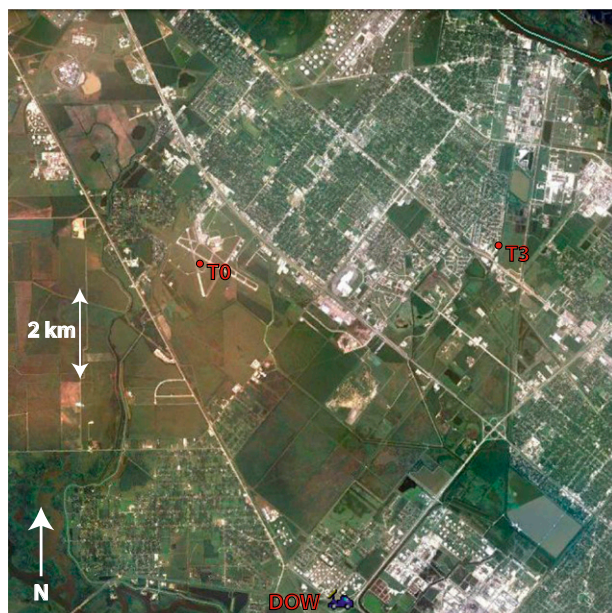
FIG. 2. Zoomed-in aerial imagery of DOW and the meteorological tower (T0 and T3) deployment in Port Arthur. Displayed area corresponds approximately to the black rectangle in Fig. 1.
